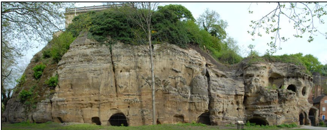
The newly cleaned south end of Castle Rock, as seen from Castle Boulevard.
